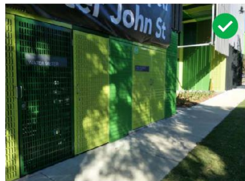
Figure 23 Harrow St Carpark, Box Hill | MGS Architects Building service cabinets are integrated into the building facade design.
