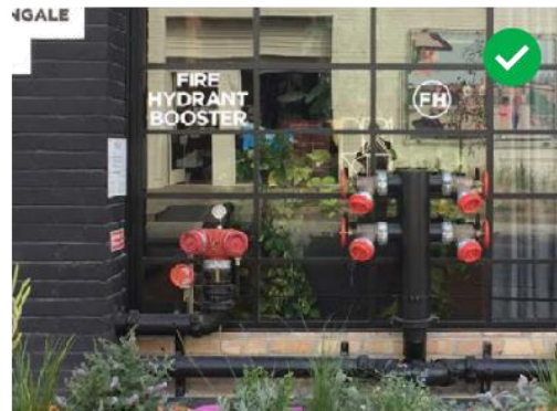
Figure 22 Nightingale 1, Brunswick | Breathe Architecture Building service elements are partially exposed to maximise clear glazing at ground level (Photo: Bonnie Herring)
