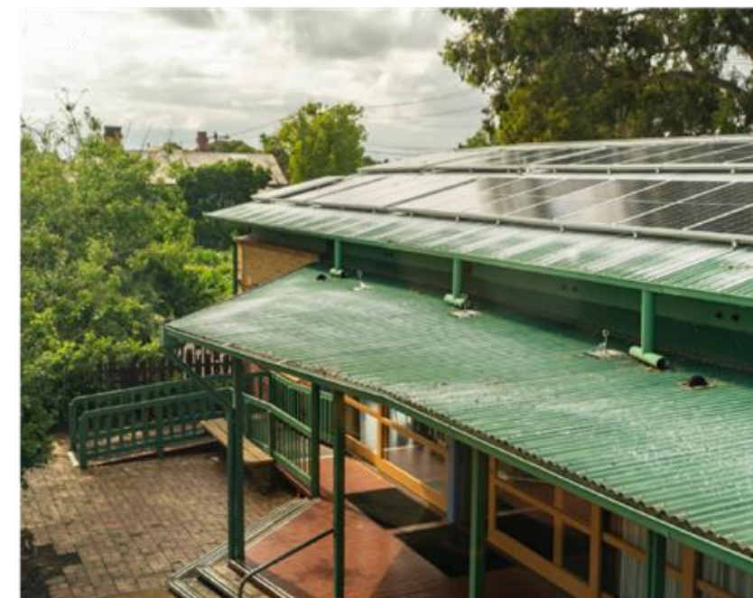
IMAGE: 15KW ROOFTOP SOLAR SYSTEM ON THE BOX HILL COMMUNITY ARTS CENTRE
