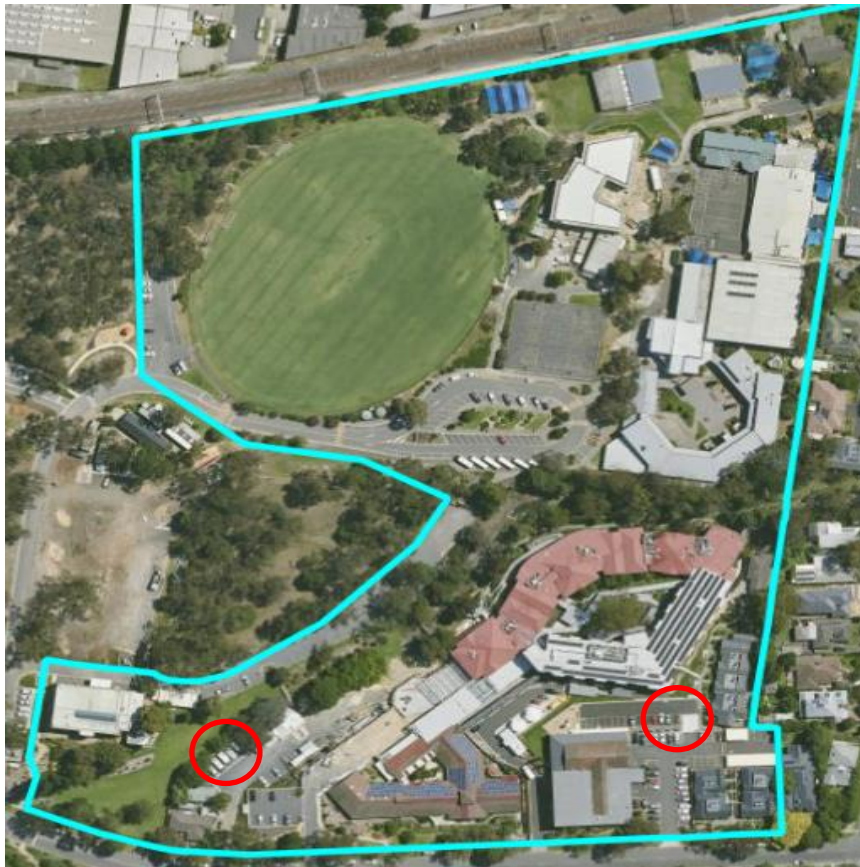
Aerial Image of subject site – Location of proposed carports circled in red.
