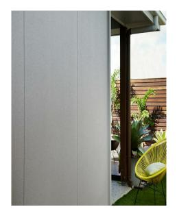
FC1 JAMES HARDIE FIBER CEMENT SHEET CLADDING EASYLAP PANEL WITH TEXTURED PAINT COLOR: DULUX SILKWORT
