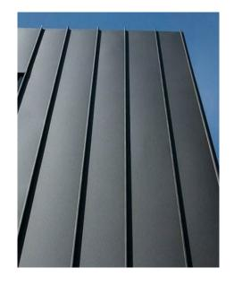
APECS 400 - SINGLE LOCK STANDING SEAM VERTICAL INTERLOCKING ALUM. CLADDING COLOUR: DULUX POWDERCOAT MONUMENT MATT
