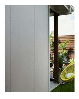
FC1 JAMES HARDIE FIBER CEMENT SHEET CLADDING EASYLAP PANEL WITH TEXTURED PAINT COLOR: DULUX SILKWORT
