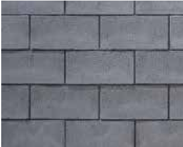
Concrete blockwork exterior walls Source: Open House
