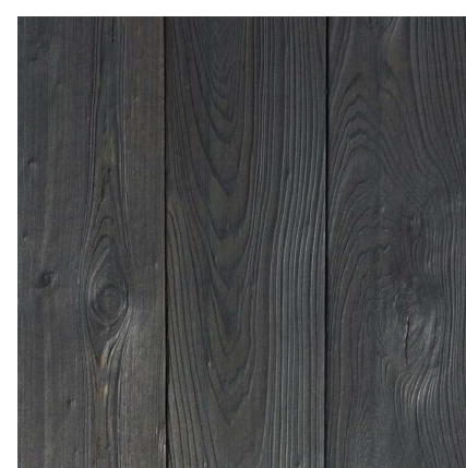
TC02 TIMBER CLAD WALL STAINED BLACK
