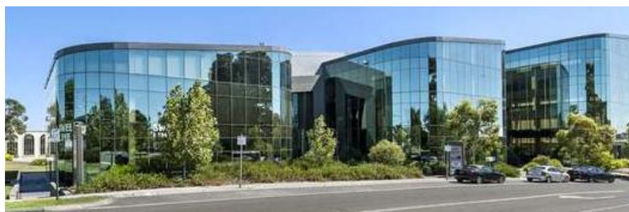
630 Mitcham Road Mitcham (Redland Estate Industrial Precinct)
