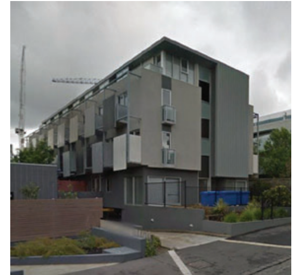
D. 8 Bruce Street 4 Levels Complete
