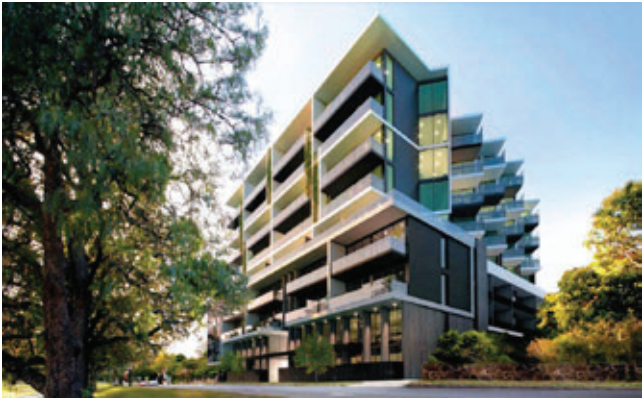
D. 5-7 Irving Avenue 9 levels Under construction
