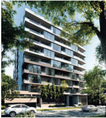
C. 15-17 Irving Avenue 10 levels Under construction
