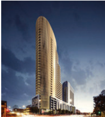
G. 850 Whitehorse Road 36, 26 levels Under construction
