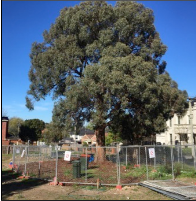
Figure 3. Install fencing around the perimeter of the TPZ.
