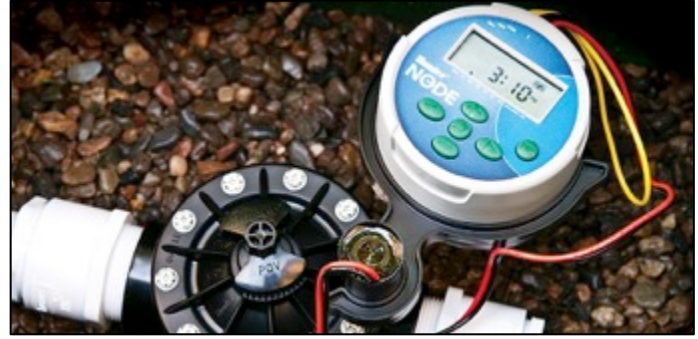
Figure 6. Automated controllers are a reliable way to regulate water quantity/frequency.
