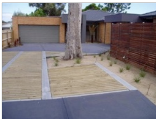
Figures 7 & 8. Bridging system within the SRZ of a canopy tree (Council of Arboriculture Victoria)
