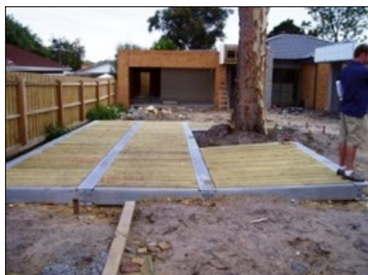
Figures 7 & 8. Bridging system within the SRZ of a canopy tree (Council of Arboriculture Victoria)
