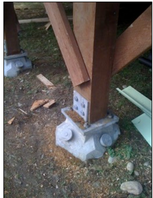
Figure 17. 'Pin' foundations are suitable for urban dwellings.
