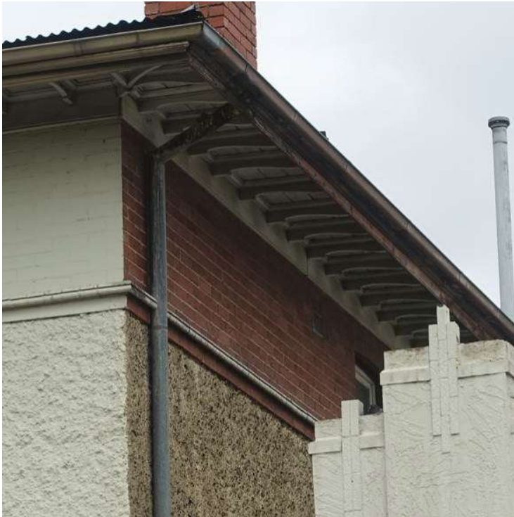
Figure 31. North-west corner of the former Railway Hotel showing unpainted tuckpointed brick and roughcast render below the eaves. (Landmark Heritage, 2022)
