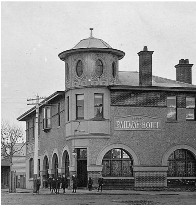
Figure 29. Stutt's Railway Hotel soon after completion of the corner section. Note the freshly tuckpointed brickwork below the eaves and in the ground-floor piers. (Detail of an image of 'Station St Box Hill', www.fletchers.net.au )
