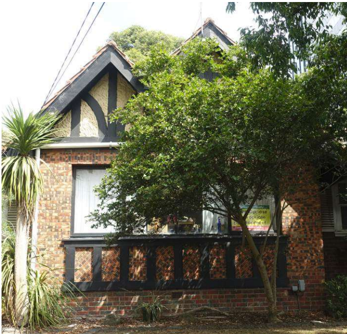
Figure 44. The two projecting front gables, with fashwerk executed in tapestry bricks below the window opening. (Landmark Heritage, 2022)
