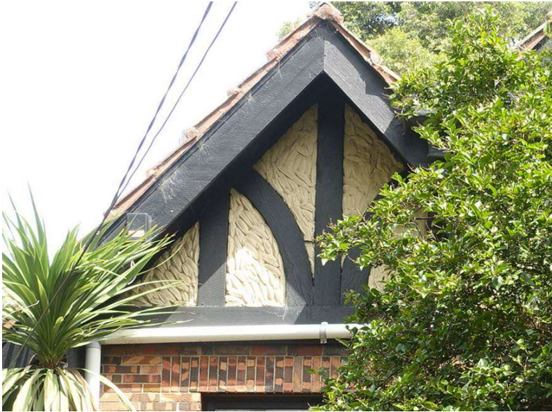
Figure 43. Detail of the textural render to the half-timbered gable and tapestry brick wall below. (Landmark Heritage, 2022)
