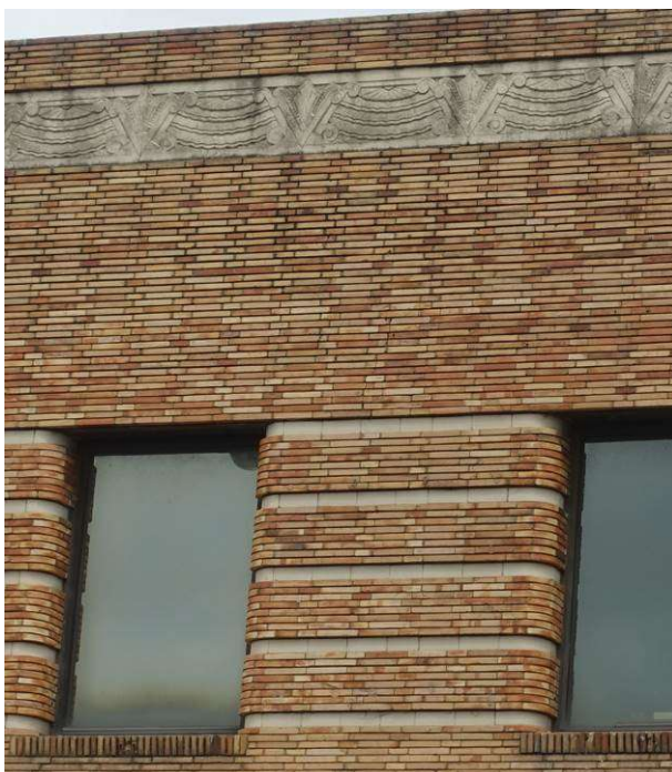
Figure 9. Detail of the first-floor brickwork and pressed-cement band. (Landmark Heritage, 2022)
